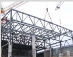
Roof Trusses in Construction
